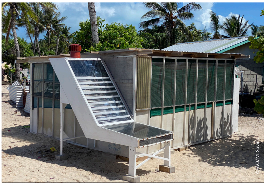
Urban fish processing facility Newerewere, Tarawa, Kiribati, 2022.
