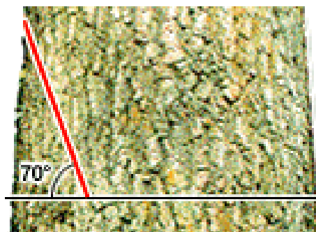
Bottom sloping cut.
