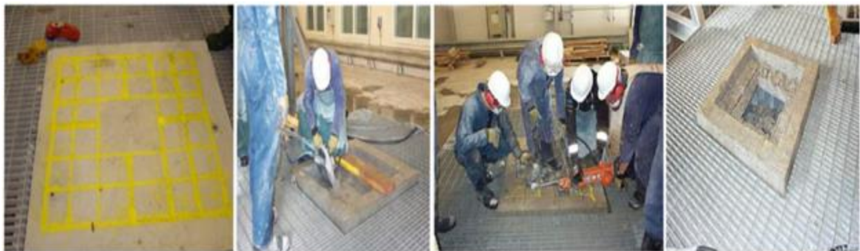
Figure 9.7. Concrete Entry Step Cut.
